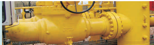
GDR-5 Pig Ball Valve / Pipeline Luncher and Receiver
